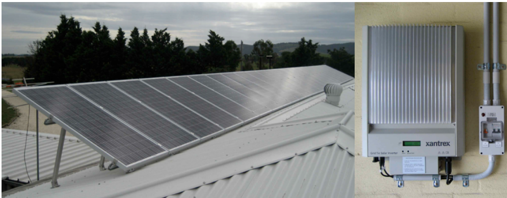
Solar panels on tilt frames to face north at 30°, Inverter to convert DC electricity to AC
